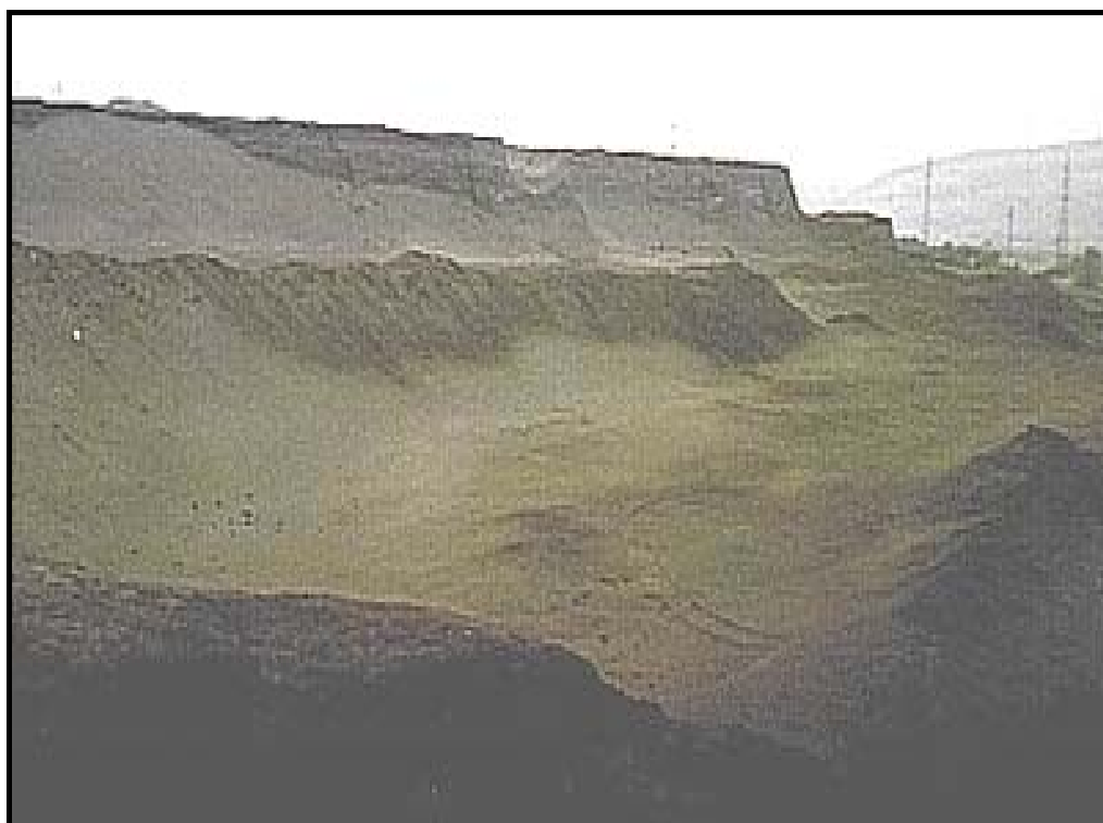
FIGURE 2. FERROUS WASTES FROM AGGLOMERATING PLANTS AND BLAST FURNACES, DEPOSITED IN PONDS
