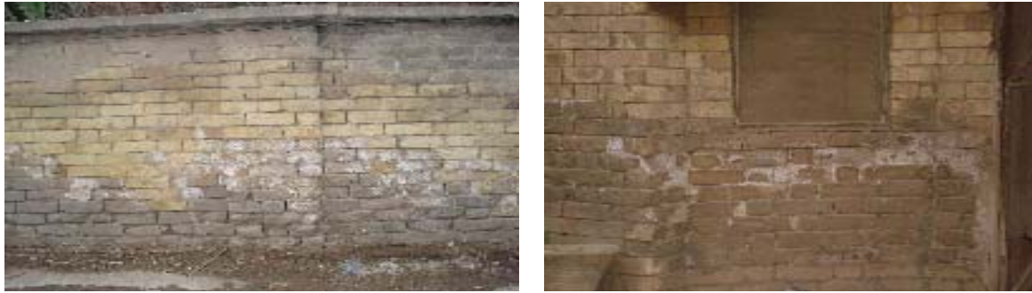
Figure 1. Traces of leached salt and deterioration in a brick fence and a bearing wall.
