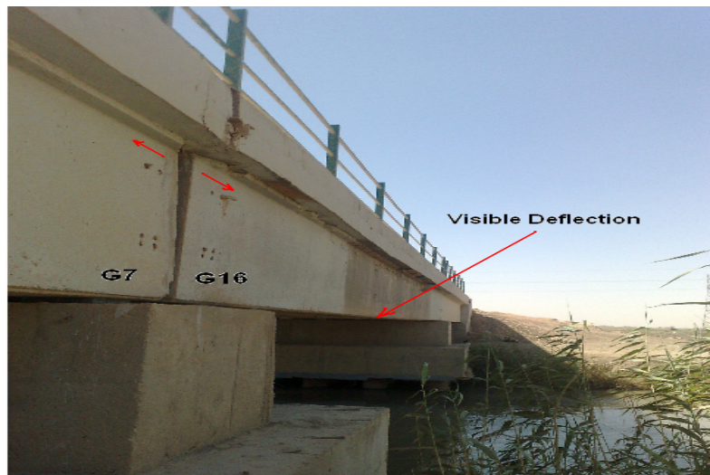
Figure 1. Visible mid span Deflection of the Intermediate Panel
