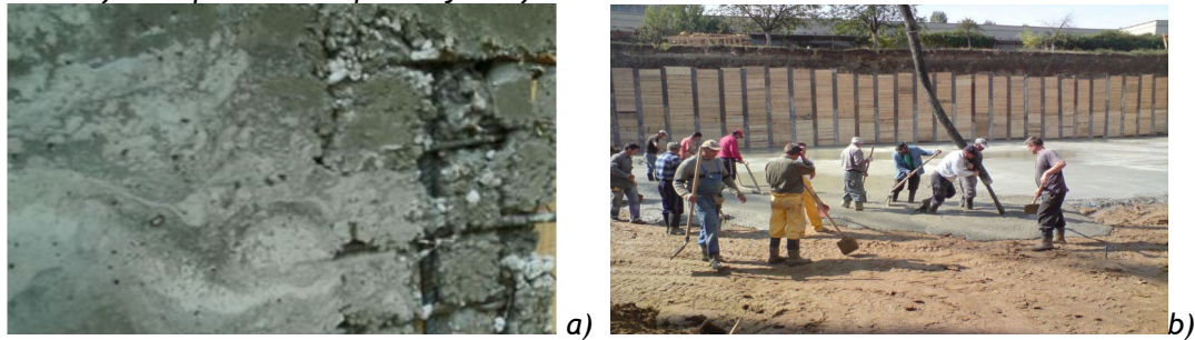
Figure 2. a) Poor compaction of a reinforced concrete column b) The huge number of workers involved in the compaction process
