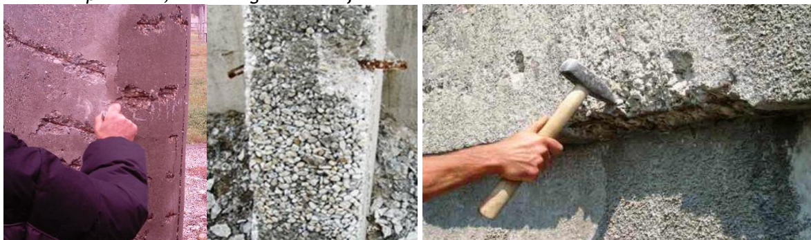
Figure 1. Poorly compacted concrete
