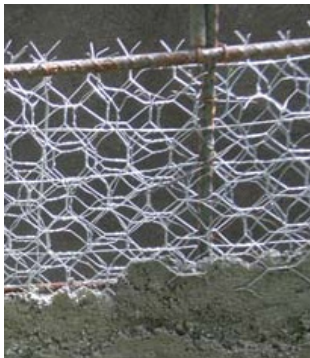
Figure 1. Ferro cement detail
