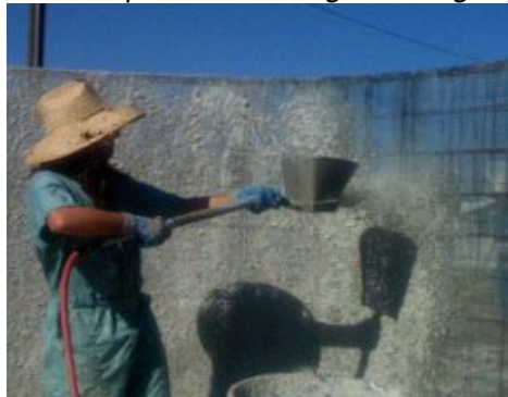
Figure 2. Applying the mortar (a), (b)
