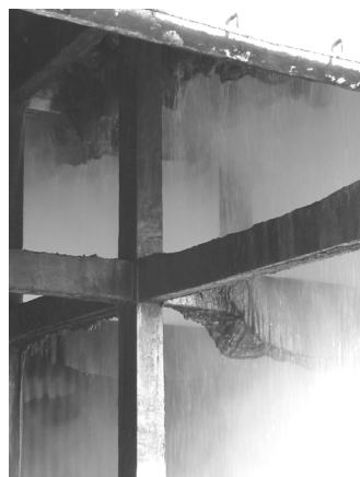
Figure 3. Incrustations in pipes and cooling towers [3]
