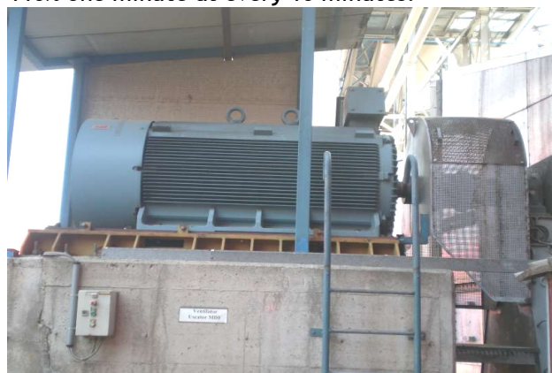
Figure 6. ABB motor of 1800 kW which moved the ventilator with J=4001 \text{ kgm}^2
