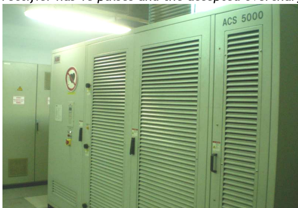
Figure 5. The panel of the ACS 5000 type converter - 2100 kVA
