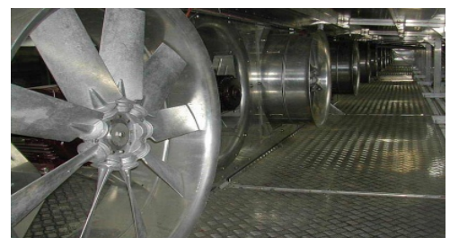
Figure 5 -Axial fans for dryers (Photograph courtesy of Eco High Tech)
