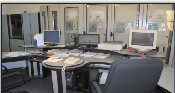
Figure 4. Control room of PS Sudrigiu Table 1. Specifications of HG and trafo from HPP Fughiu and Săcădat
