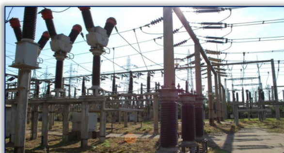
Figure 5. External devices from 110 kV of PS-CET I Table 2. Specifications of HG and trafo from HPP Lugașu and Tileagd
