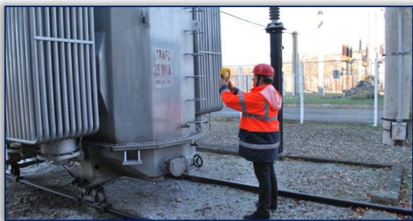
Figure 2. Set transformer from HPP Tileagd
