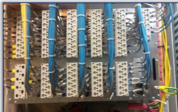
Figure 9. Cover protection equipment earthed
