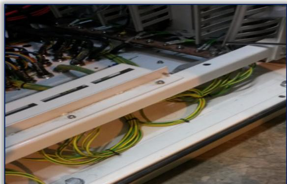
Figure 8. Sample for protection panel earthed
