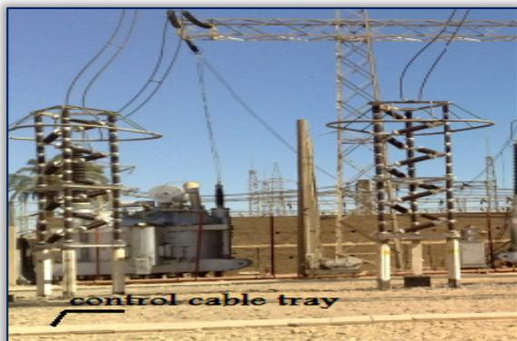
Figure 7. Control cable trays in substation
