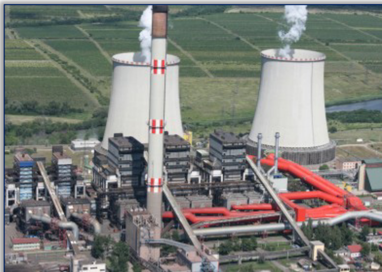
Figure 1. Mátra Power Plant
