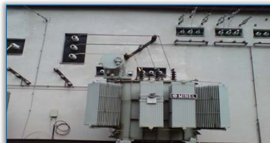
Figure 1: Transformer connected to the electrical grid in substation 35/10 kV [1]
