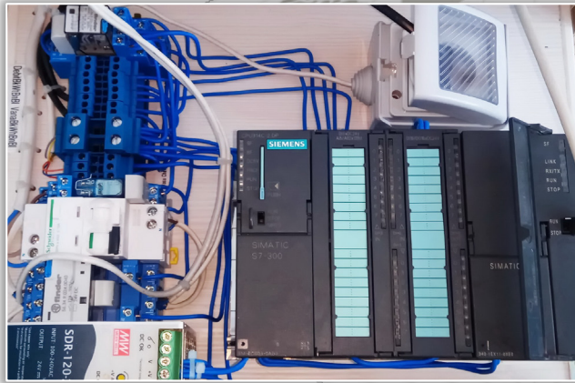
Figure 2. PLC wired into the system
