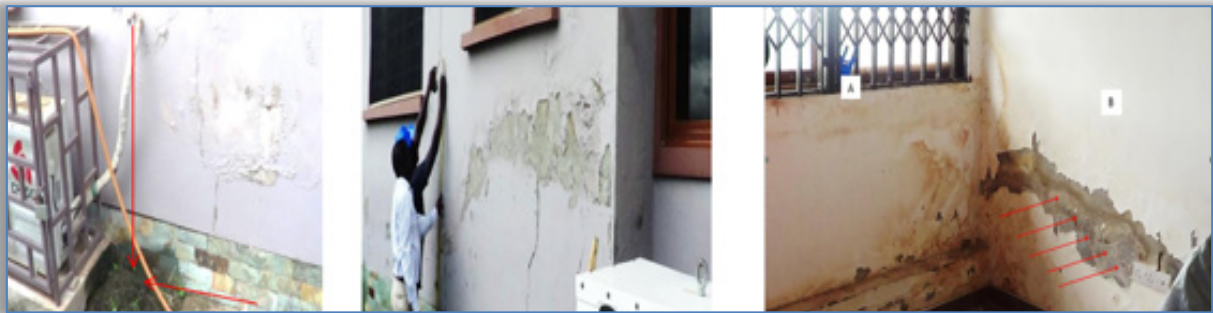
Figure 5a. Some symptoms of dampness identified from the building in Case 3 (Source: [24])
