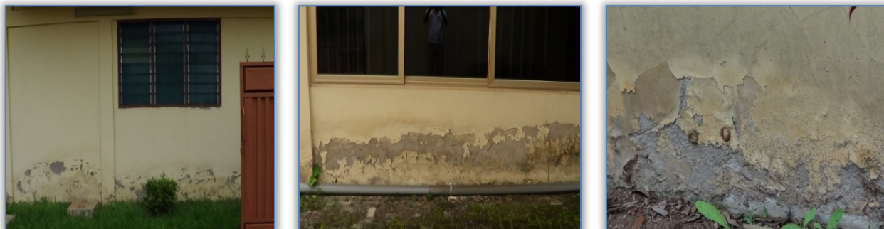
Figure 3a. Some symptoms of dampness identified from the building in Case 1 (Source: [22])
