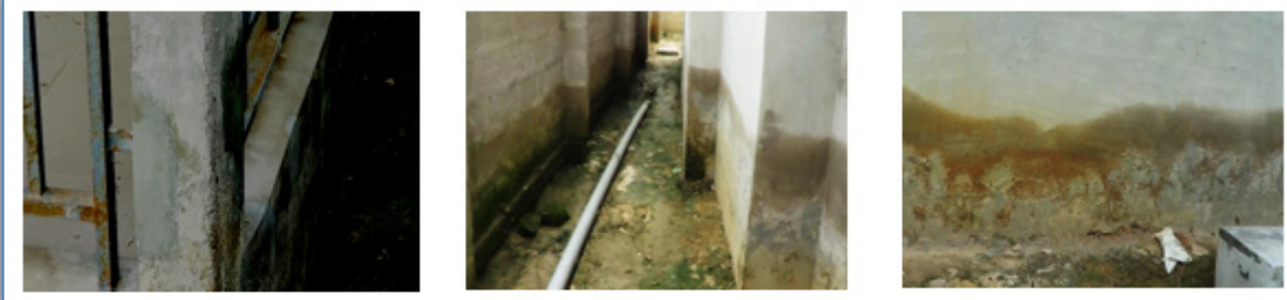
Figure 4a. Some symptoms of dampness identified from the building in Case 2 (Source: [23])
