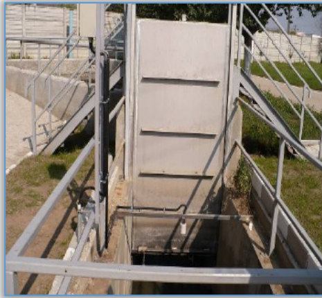
Figure 3. Taking the waste water out of sewers – the water enters into the mechanical stage
