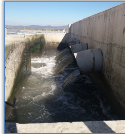
Figure 4. Waste water discharge, mechanically cleaned
