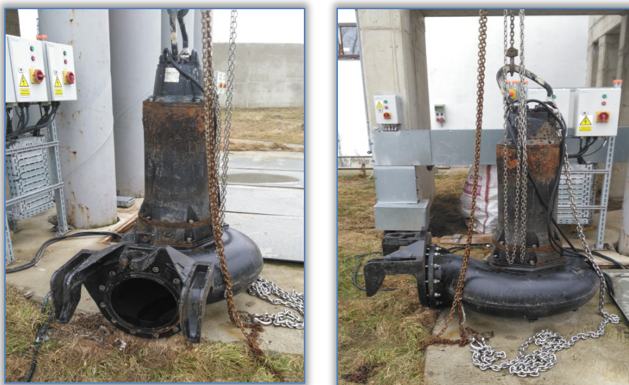
Figure 2. Pump designed for domestic waste water discharge
