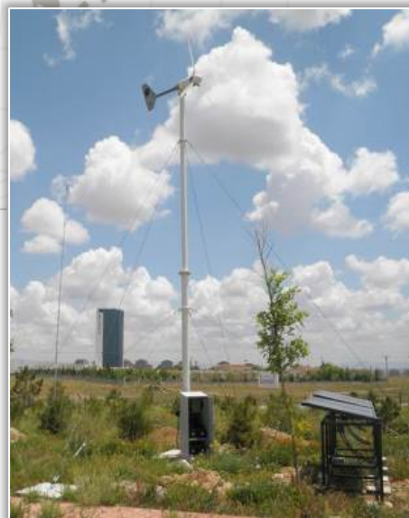
Figure 2. PV-wind based hybrid power plant in the garden of Konya Selcuk University Technology Development Zone
