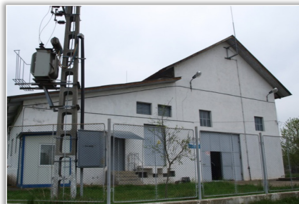
Figure 11. Micro –hydro Plant Nimăeşti
