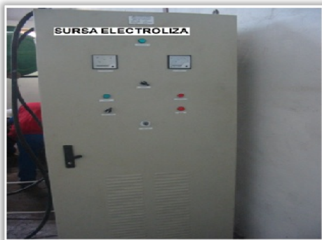
Figure 2. DC power supply for electrolysis supply of ZnSO_4 solution for metal zinc extraction
