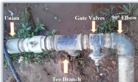
Figure 5: Fittings of a network link at HAC Farm
