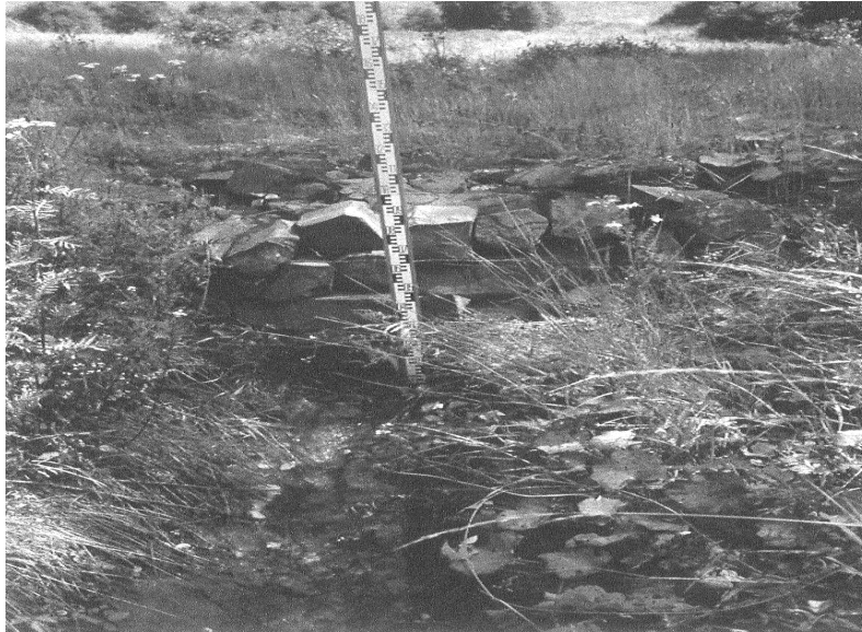
Fig.6. Rubble drain in the base of dump
