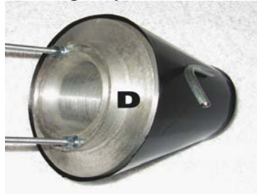
Figure 11. The internal diffuser
