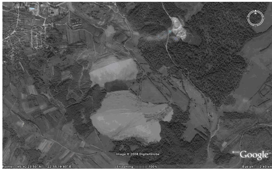
Figure 3. The integration plan in sludge bed no.2 and 3, Teliuc area
