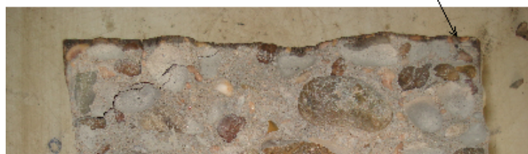
Fig. 4. Wax penetration inside the top surface of concrete
