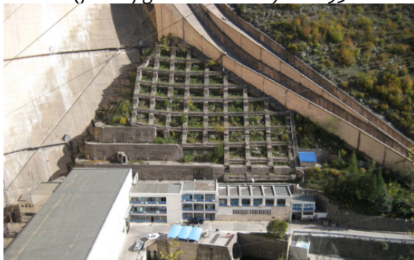
Figure 1: Field of ground anchors Grncarevo Hydroelectric Power Station
