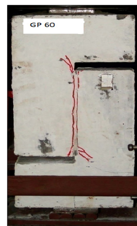
Figure 7. Crack pattern in reinforced push-off specimen GP60
