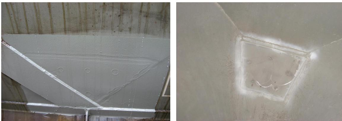
Figure 6. Crack repair on the tanks
