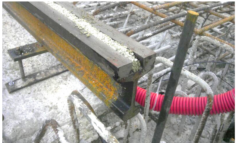
Figure 5 – Connection of rails with armature
