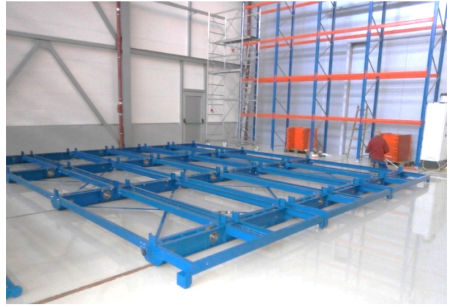
Figure 8 – Mounted undercarriage of the movable racks
