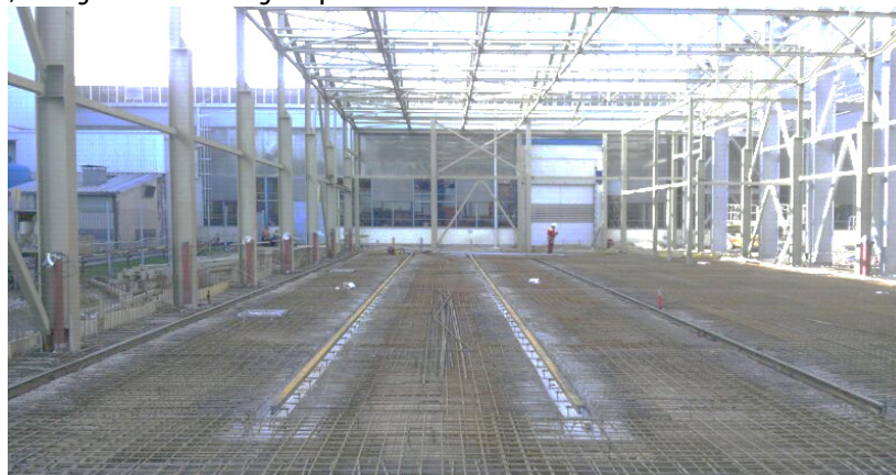
Figure 6 – Armoring plate with rails
