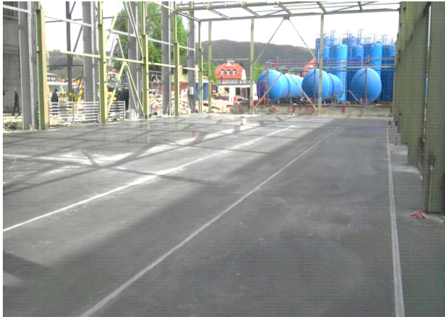
Figure 7 – Concrete plate with rails
