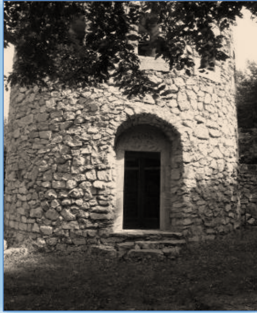
Figure 2. A section of walling from uncarved tones. (View of the rotunda from the entrance.)
