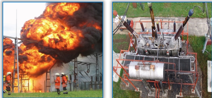
Figure 9. Results of an uncontained transformer fire
