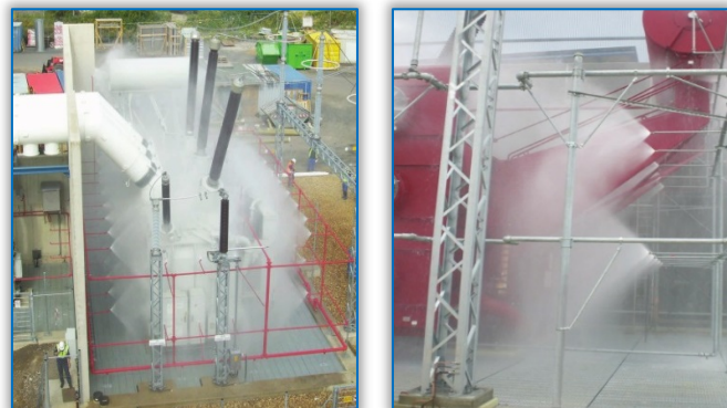
Figure 10. Transformer equipped with firefighting system
