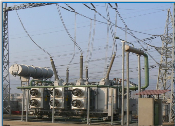
Figure 1. Power transformer in high voltage power station
