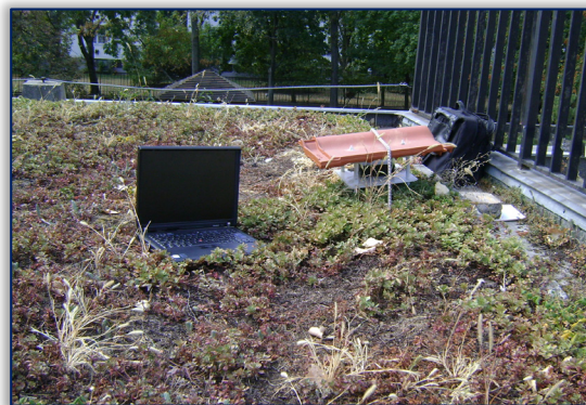
Figure 1. Green roof and terraced roof with the measuring unit
