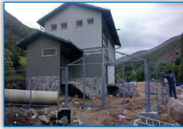
Figure 5. Setting up a structure for stacking the panels for noise protection
