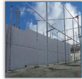
Figure 5. Setting up a structure for stacking the panels for noise protection
