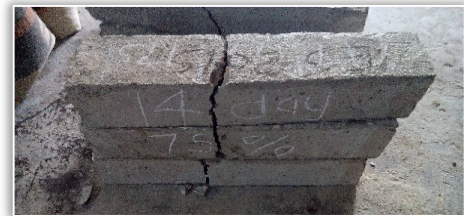
Figure 5-Failure Mode of Concrete Beam
