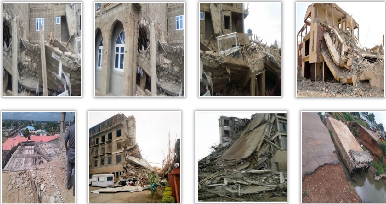
Figure 1: Some collapsed buildings in Ilorin (2017-2018). Source: Nigerian Society of Engineers, Ilorin Branch, 2019)
