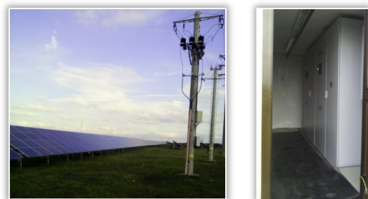
Figure 5 - Images with Salonta PVP: a - for ensemble; b - inside inverter box (conversion unit)
