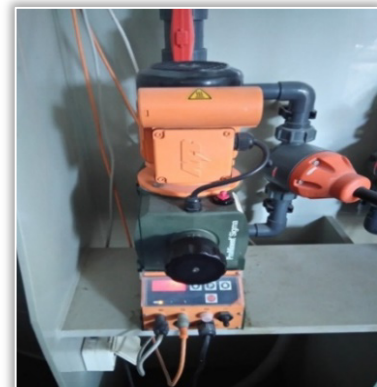
Figure 4. Dosing pump type: Prominent
