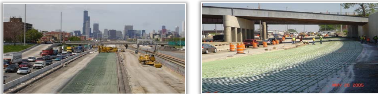
Figure 1: Continuously reinforced concrete pavement under construction
