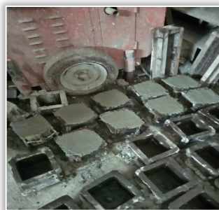
Figure 1. Casting of cubes for compressive strength
