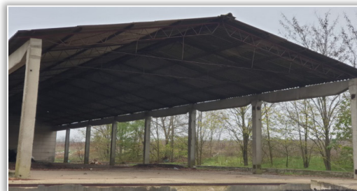
Figure 6 – Semi-open storage area
