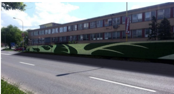
Figure 10. East Slovak printer with designed Durisol noise barrier (Building 1)
