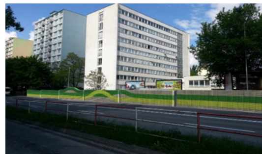
Figure 11. District office of Kosice with the proposed noise barrier wall Durisol (Building 2)
