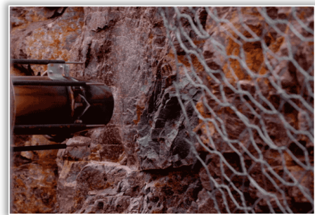
Figure 2. Petra’s “Swiftly” robot heats and grinds the hardest stone on Earth, without touching it [14, 15].
