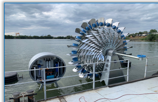
Figure 8 – The assembly of the 2 devices for taking over and treating water from the Danube through filtration
