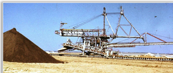
Figure 3 – Land reclamation process and soil storage in the day surface
