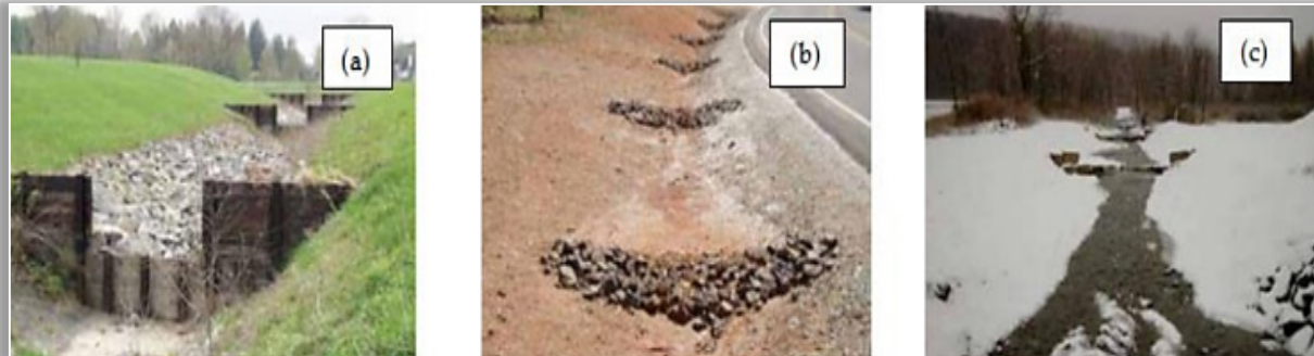
Figure10. Different types of Check dams, (a) Wooden check dam, (b) Rock-filled check dam, and (c) Stone check dam [21]
