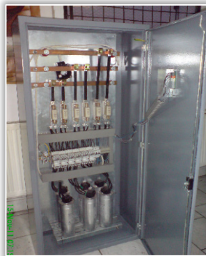
Figure 3. a. The electric box with PFC (on the front side); b. capacitors banks installed in PFC
