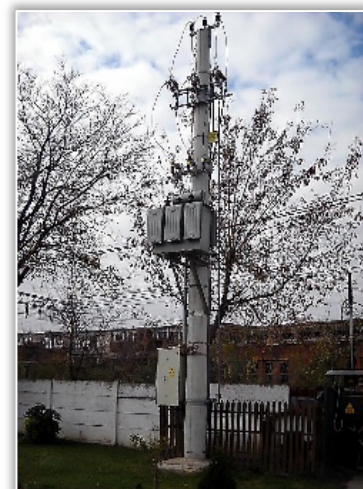
Figure 4. Low-voltage power substation placed outside from textile plant
