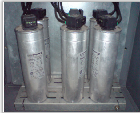
Figure 3. a. The electric box with PFC (on the front side); b. capacitors banks installed in PFC
