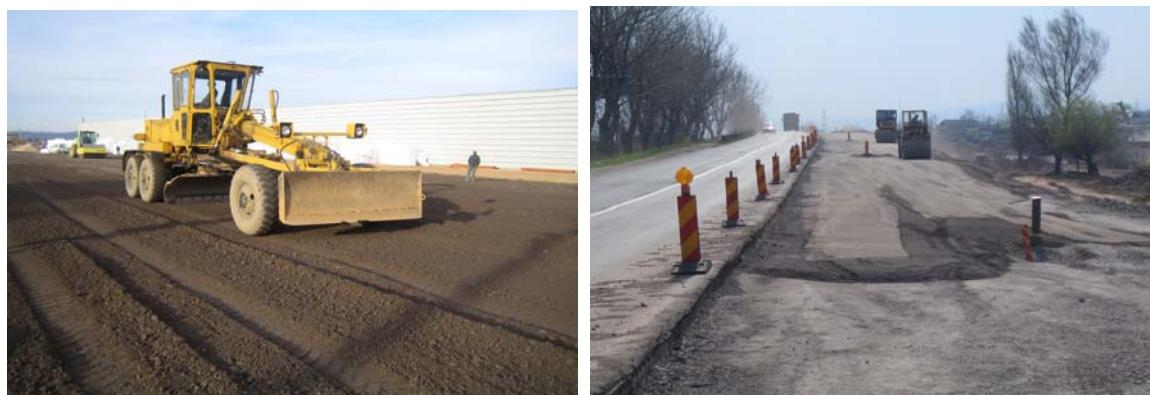
Figure 8. Slag road construction; Hunedoara - Deva
