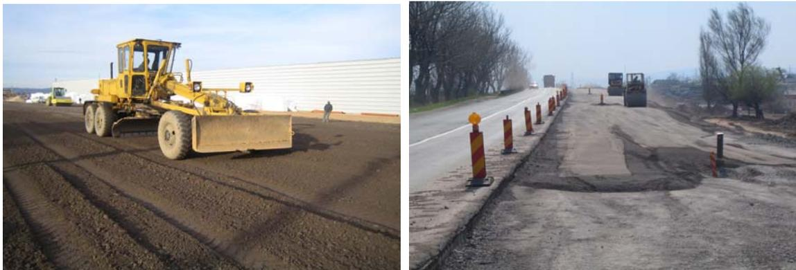
Figure 8. Slag road construction; Hunedoara - Deva
