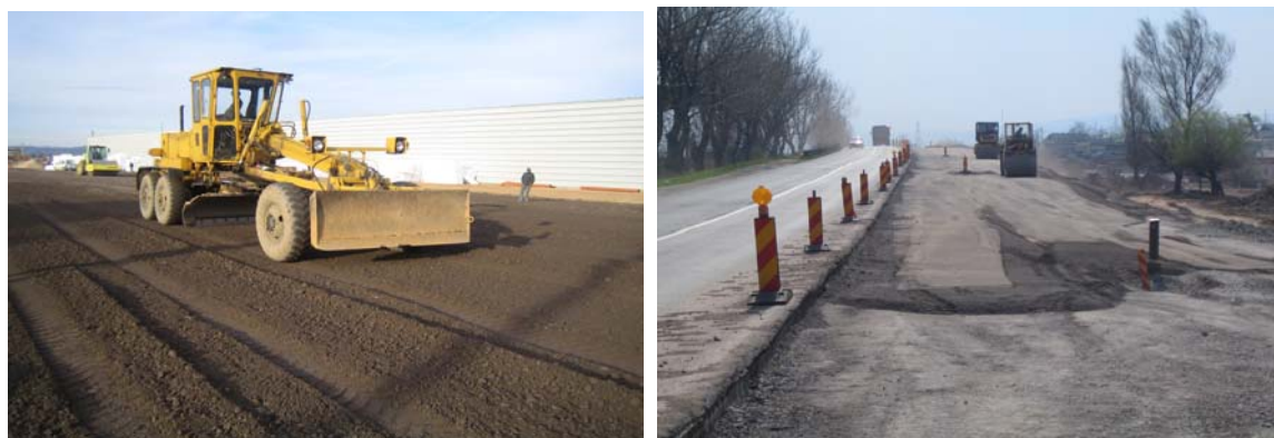
Figure 8. Slag road construction; Hunedoara - Deva
